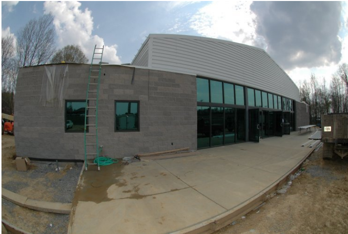
The new Merle Travis Music Center under construction
